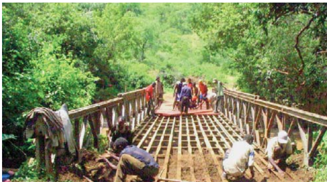
The old Kulfo Bridge in Nech Sar has been entirely renovated.
