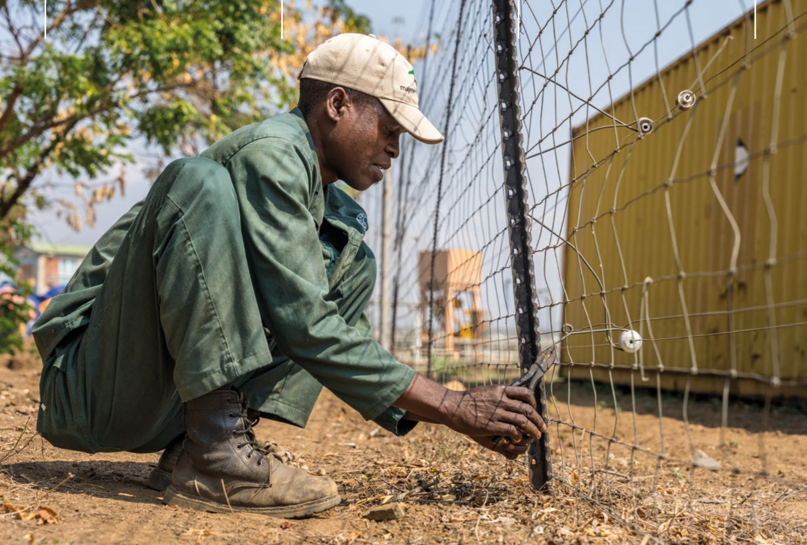
Above: Full-time fence technicians maintain the predator and elephant-proof boundary fence, Majete Wildlife Reserve, Malawi © Marcus Westberg
